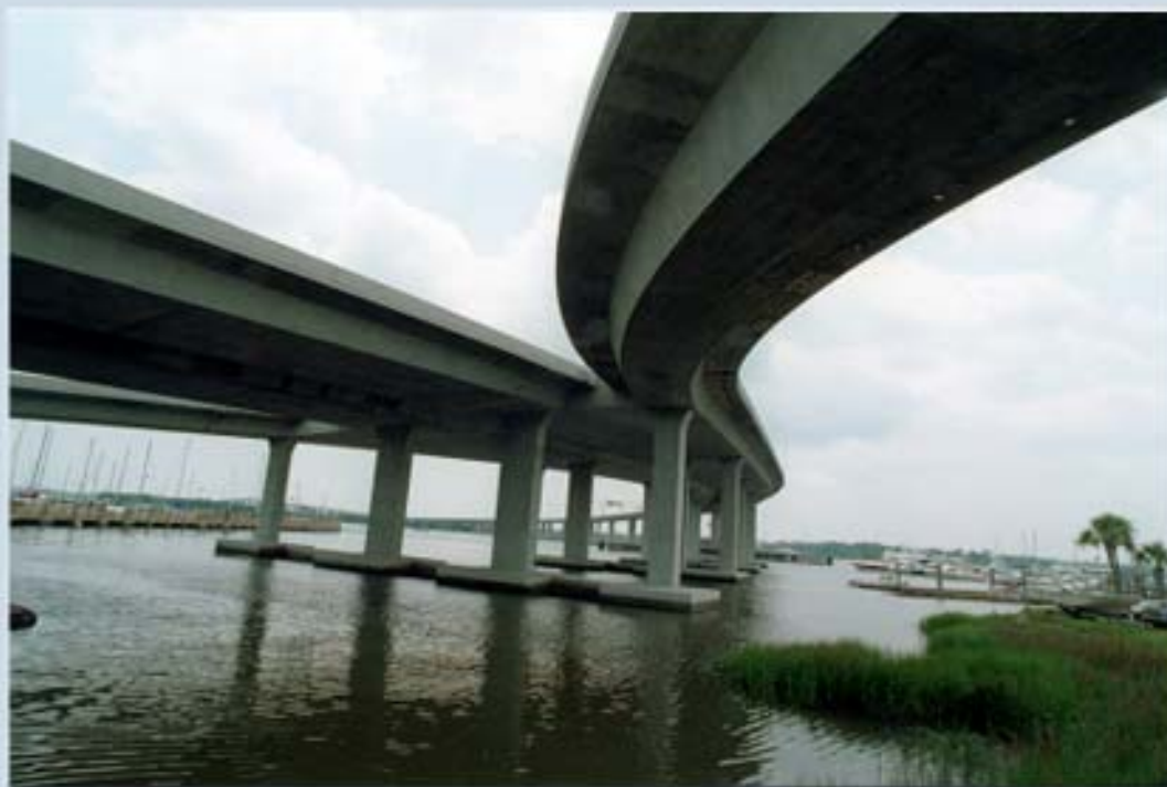
The James Island Bridge James Island, South Carolina
