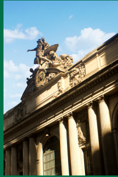
Grand Central Terminal Built 1907
