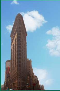
Flatiron Building Built 1902
