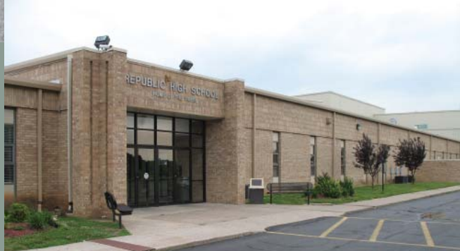
Pictured at right is the current Republic High School.
