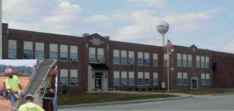
Pictured at left is the original Clever High School, built in 1929. It now houses upper elementary students, grades 4 and 5.
