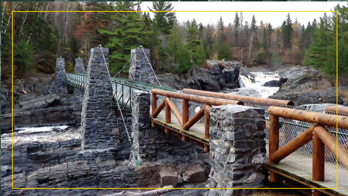
Swing Bridge, Jay Cooke State Park
