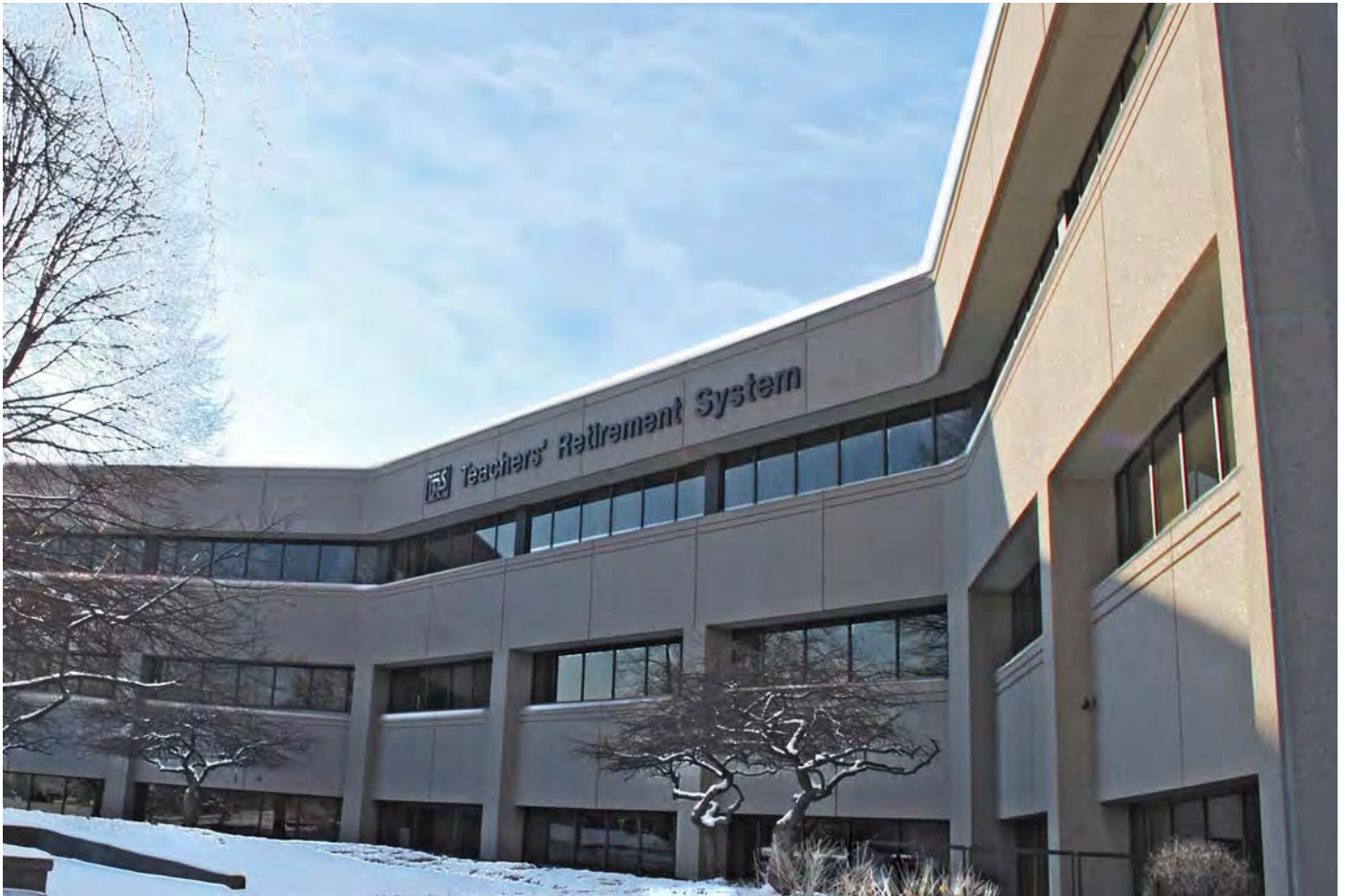
TRS Springfield office building, 1979 - present
