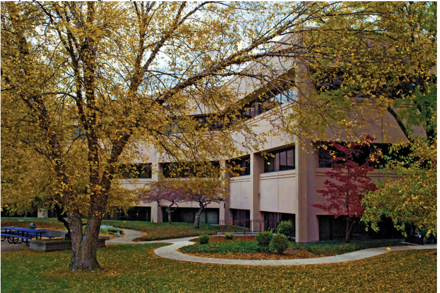
TRS Springfield office building, 1979 - present
