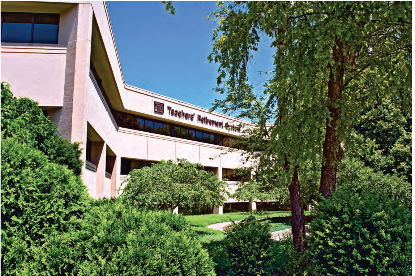
TRS Springfield office building, 1979 - present
