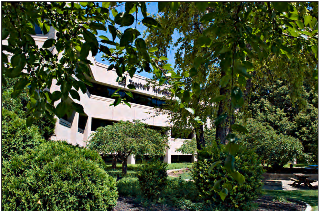
TRS Springfield office building, 1979 - present
