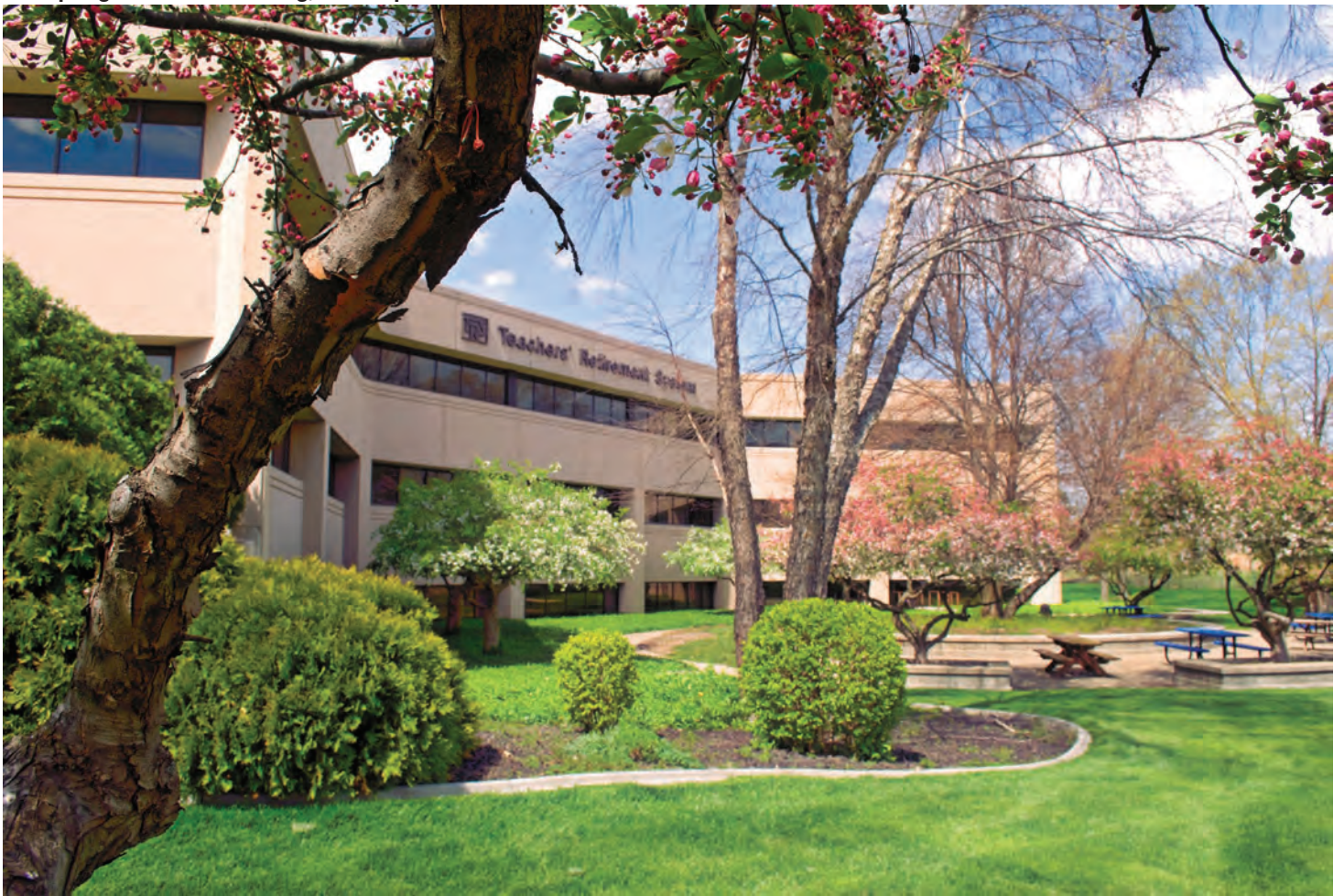
TRS Springfield office building, 1979 - present
