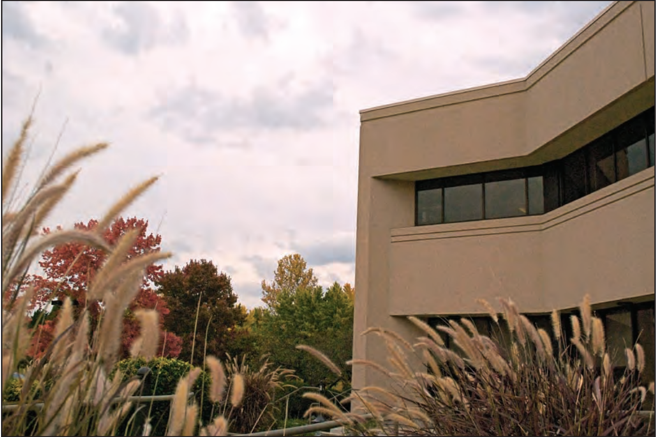
TRS Springfield office building, 1979 - present
