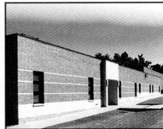
Riverton Elementary School Riverton
