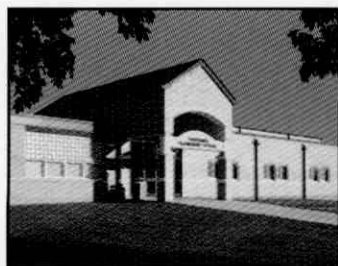
Centennial Elementary School Polo
